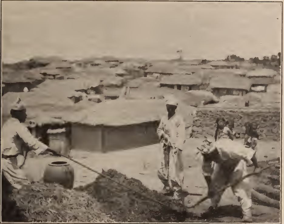
A THREE MAN POWER "STEAM" SHOVEL IN CHOSEN One man guides and two pull on the ropes attached to the shovel
